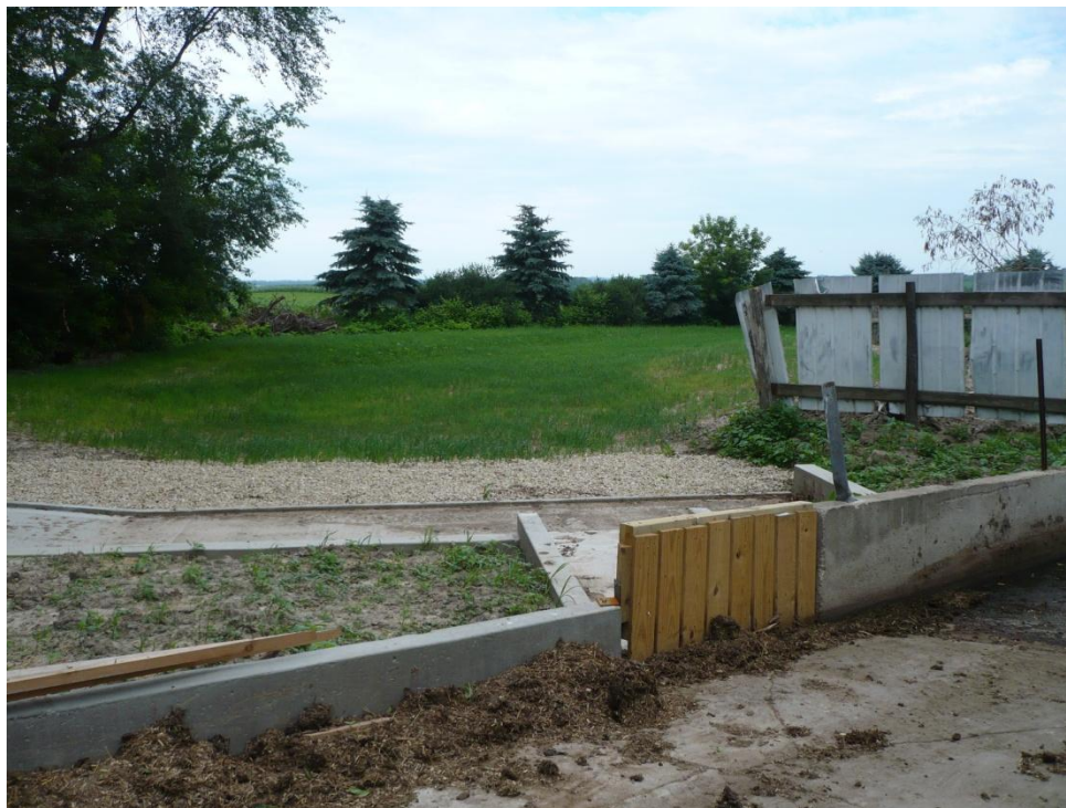
Liquid leveler, solids filter, vegetated filter strip
